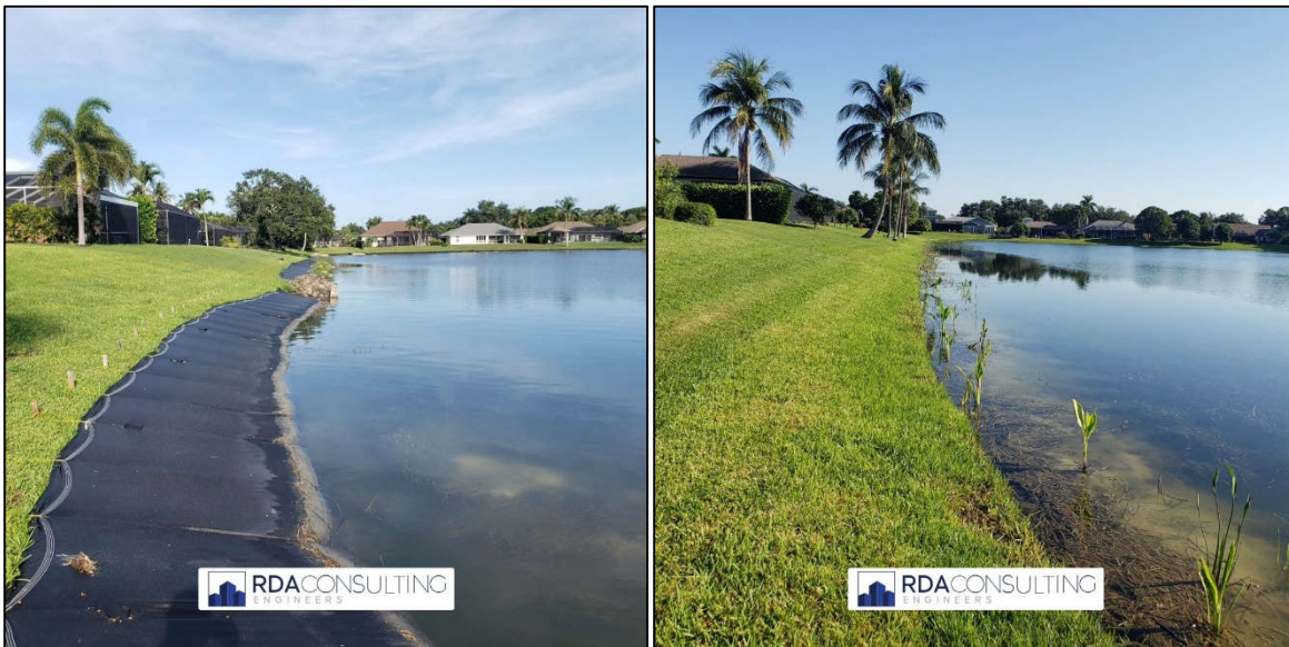
Figure 5. Erosion Control Wraps During and After. (RDA Consulting Engineers, 2026).
