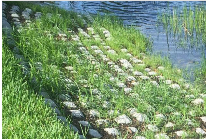
Figure 3. Vegetated Concrete Mat, Flexamat. (Seabreeze Erosion Solutions, n.d.)
